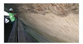
**Hidden defect:** Concrete delamination and corroded reinforcement
