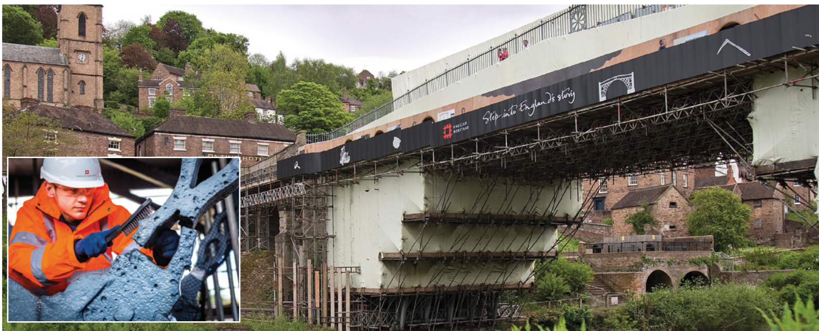
Although the bridge was fully enclosed for the refurbishment work, a walkway built alongside let visitors observe work through special portholes. Inset: detail of one of the iron members
