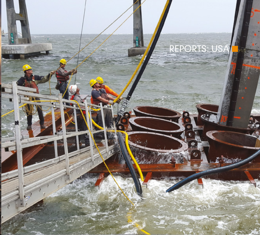
The piles were installed by a combination of jetting and driving
