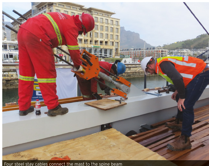
Four steel stay cables connect the mast to the spine beam
