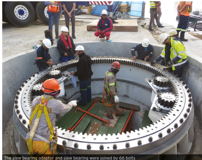
The slew bearing adaptor and slew bearing were joined by 66 bolts
