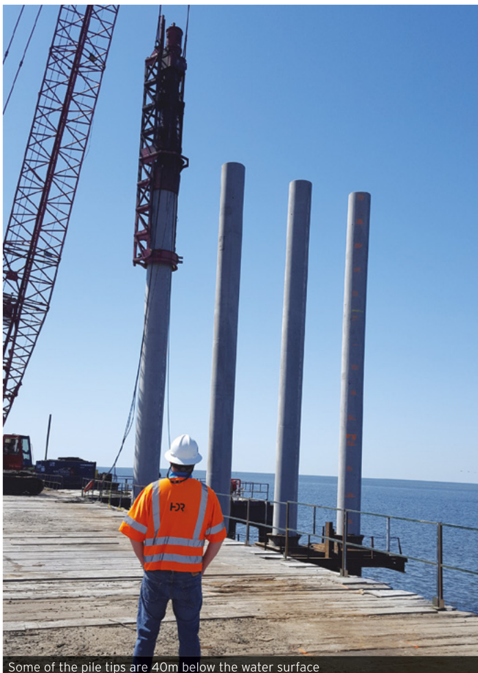
Some of the pile tips are 40m below the water surface
