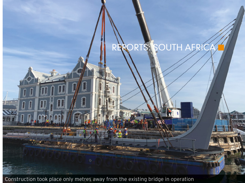
Construction took place only metres away from the existing bridge in operation
