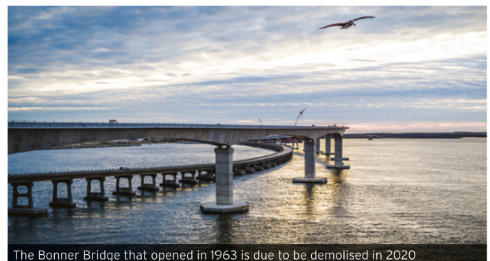
The Bonner Bridge that opened in 1963 is due to be demolished in 2020
