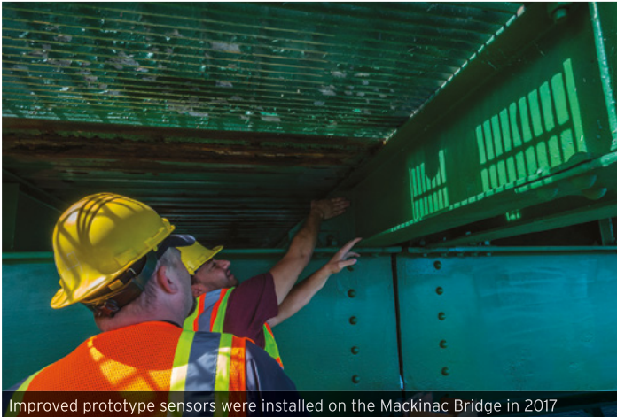
Improved prototype sensors were installed on the Mackinac Bridge in 2017
