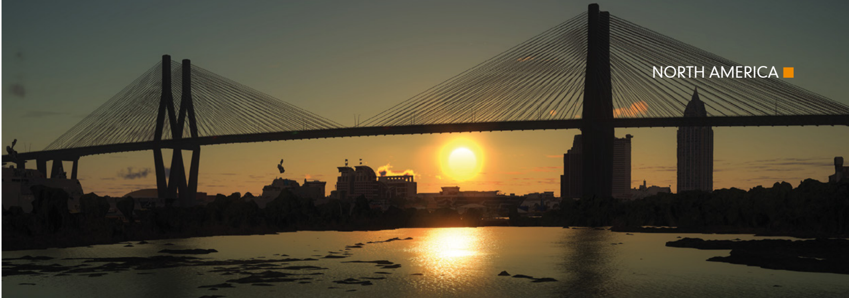
The new crossings of the Mobile River Bridge and Bayway expansion project will be managed under a 55-year concession agreement
