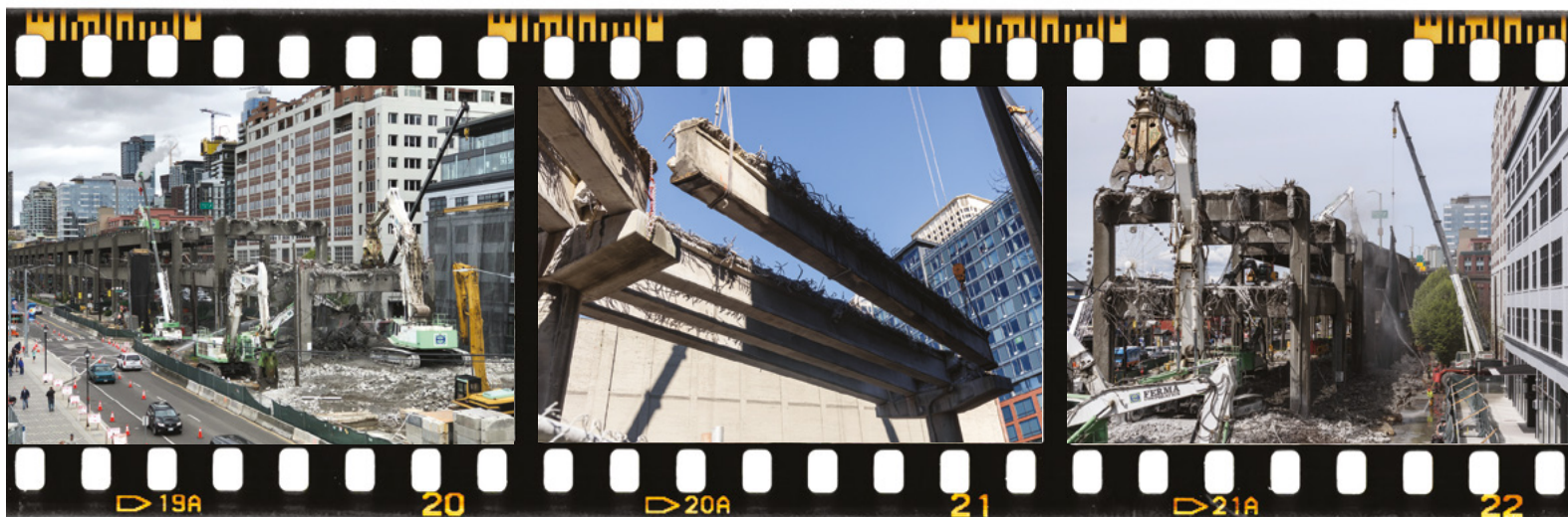
Below, left to right: the Colman Dock ferry terminal offers one of the best views as crews work their way along the waterfront. Cranes remove a girder from a section of the old Columbia Street on-ramp to southbound SR 99. Looking north from the Marion Street pedestrian bridge (images: WSDOT)
