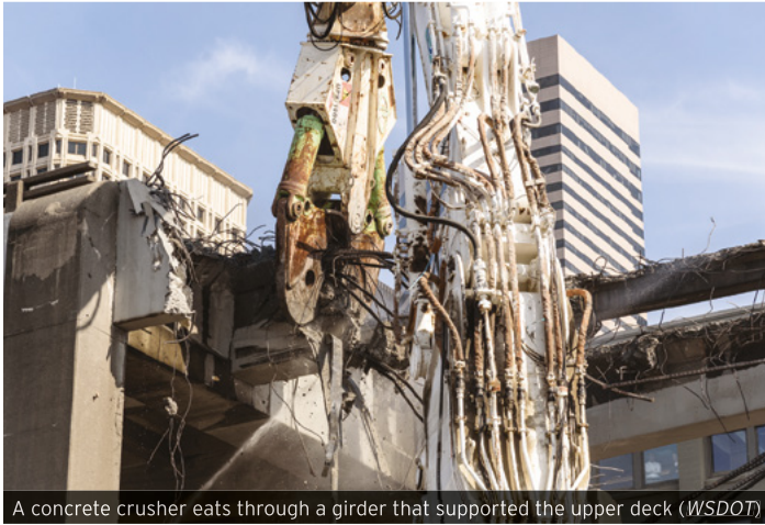
A concrete crusher eats through a girder that supported the upper deck (WSDOT)
