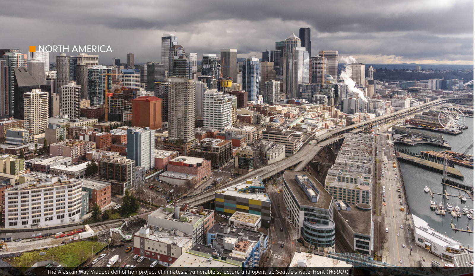
The Alaskan Way Viaduct demolition project eliminates a vulnerable structure and opens up Seattle's waterfront (WSDOT)
