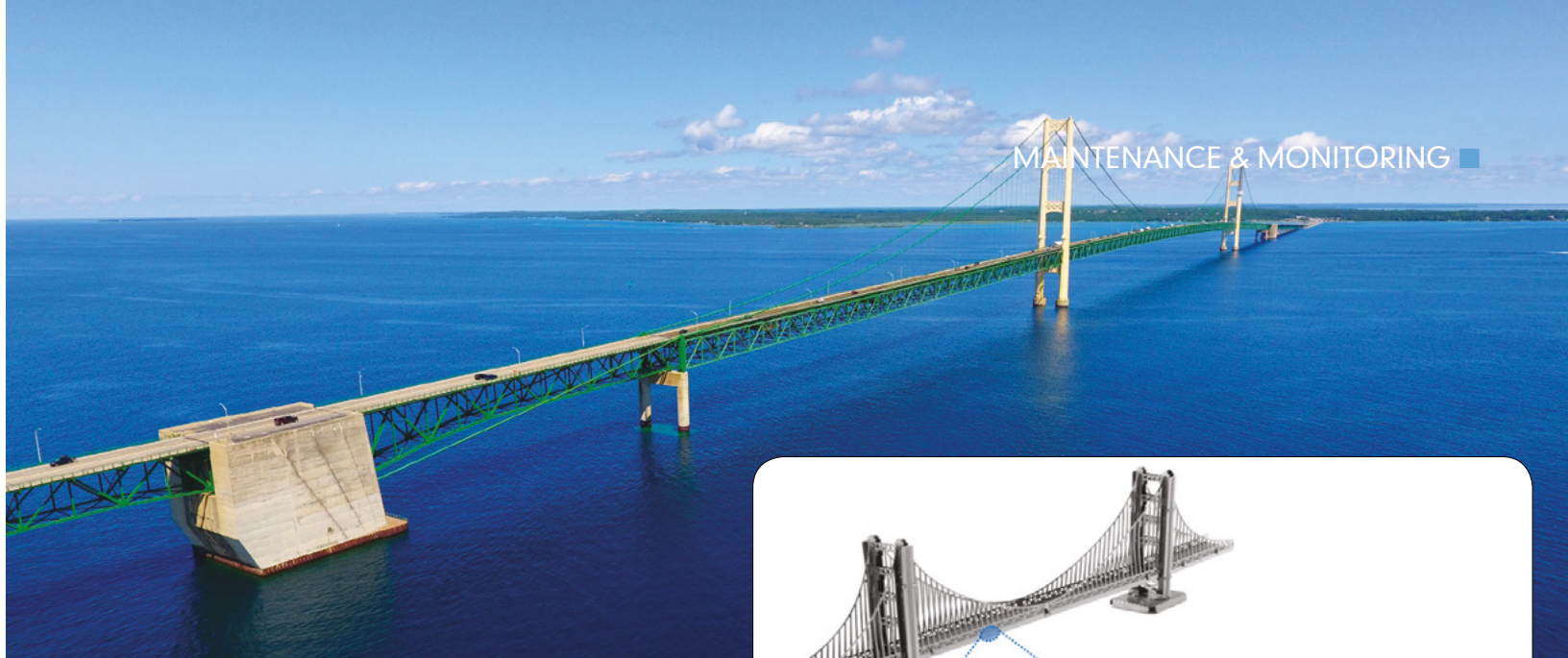
The Mackinac Bridge has hosted various sensing technologies since 2016. Inset: AI-based, damage-identification algorithms in development will isolate potential hot spots
